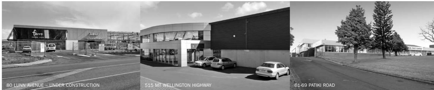
80 LUNN AVENUE – UNDER CONSTRUCTION
