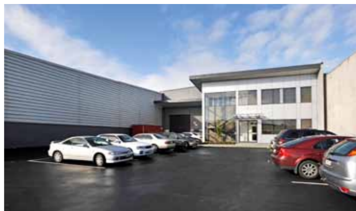
Development project: Office/warehouse for Brewcraft in North Harbour.
